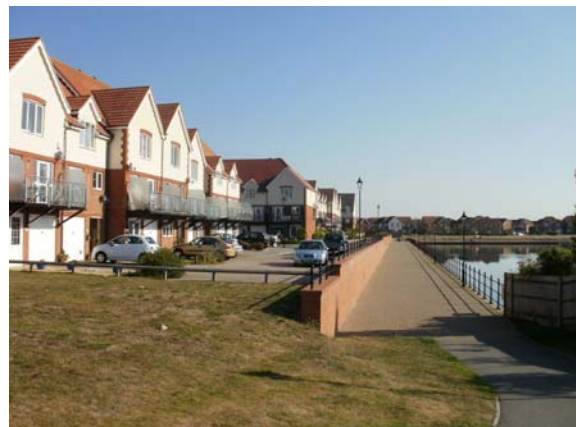
Figure 2 Housing at Brisbane Quay
