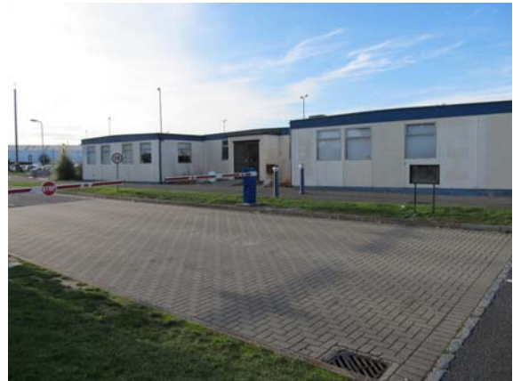
Figure 23 Portacabin Offices currently occupying Site 5
